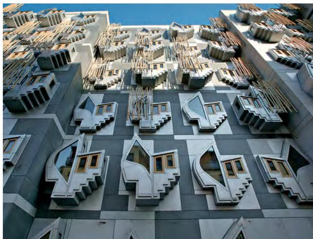
Stainless steel was used not only in the interior, but also, as grade EN 1.4404 steel sheet, for a range of external applications. The projecting windows, 50 cm and 1 m deep, on the west façade of the MPs building are clad with bent sheet. Angled and
